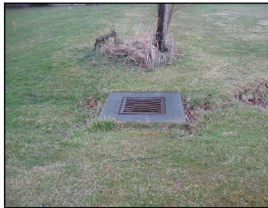
WEST SIDE SR 60 CB TO DITCH ALONG SR 60 NORTH
