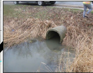
EAST SIDE SR 60 DITCH TO 30" CULVERT UNDER SR 60
