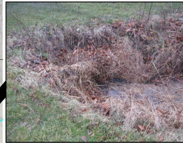
WEST SIDE SR 60 DITCH ALONG RES. #3503
