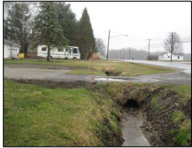
WEST SIDE SR 60 DITCH ALONG SR 60 NORTH
